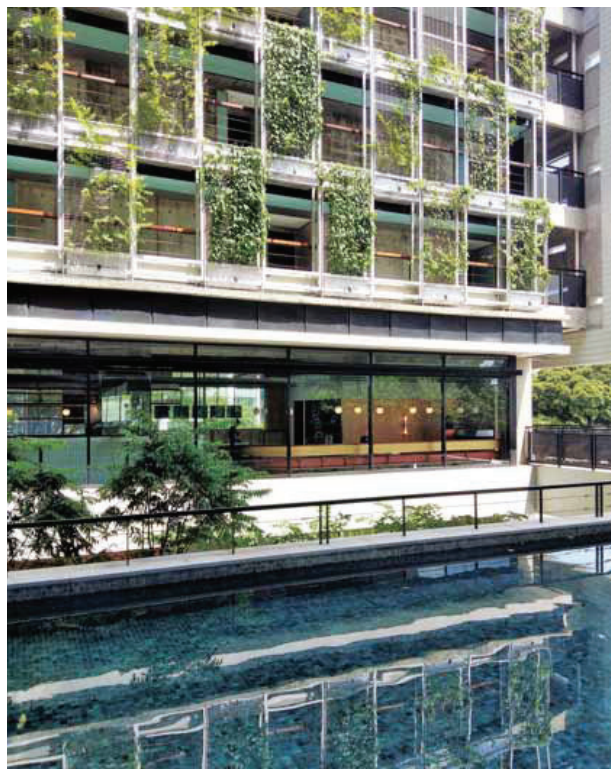
KLoé Hotel features open corridors and black aluminium cladding with vertical sun-shading fins to block out heat
